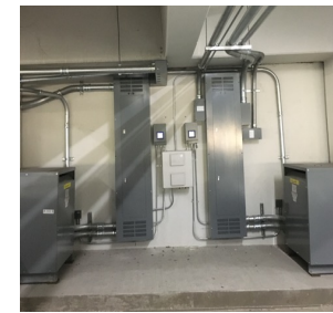
transformer & subpanels
