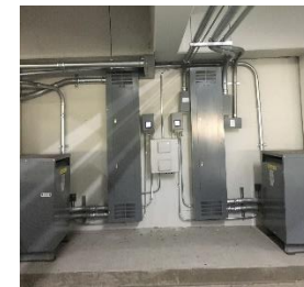
transformer & subpanels
